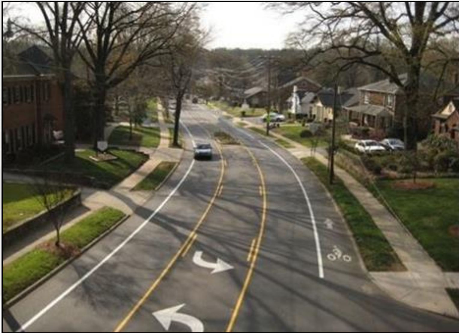
NH Route 108 Complete Streets Improvements
